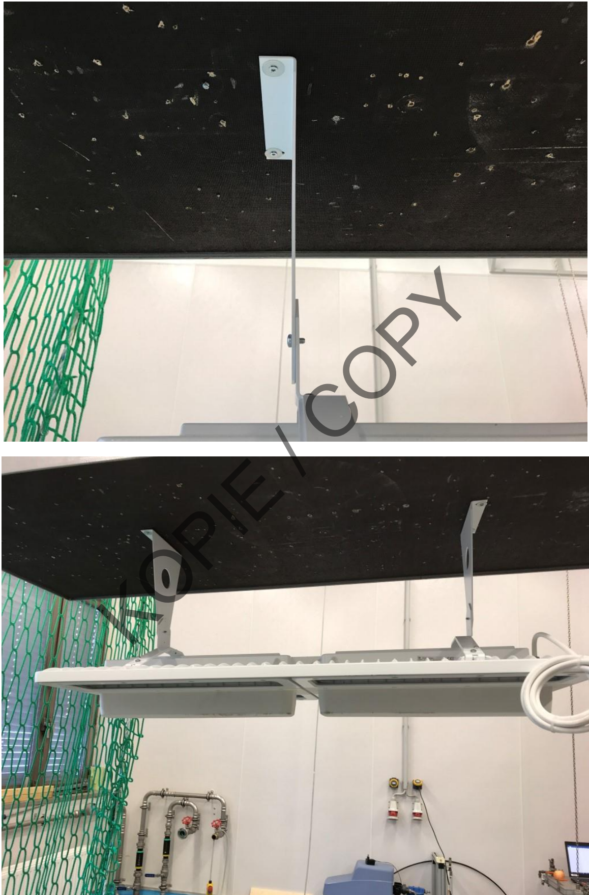
Picture 7: CR2PL L35k-840 PC WB MWCF SP WH – ceiling mounting, on AD/AW set
